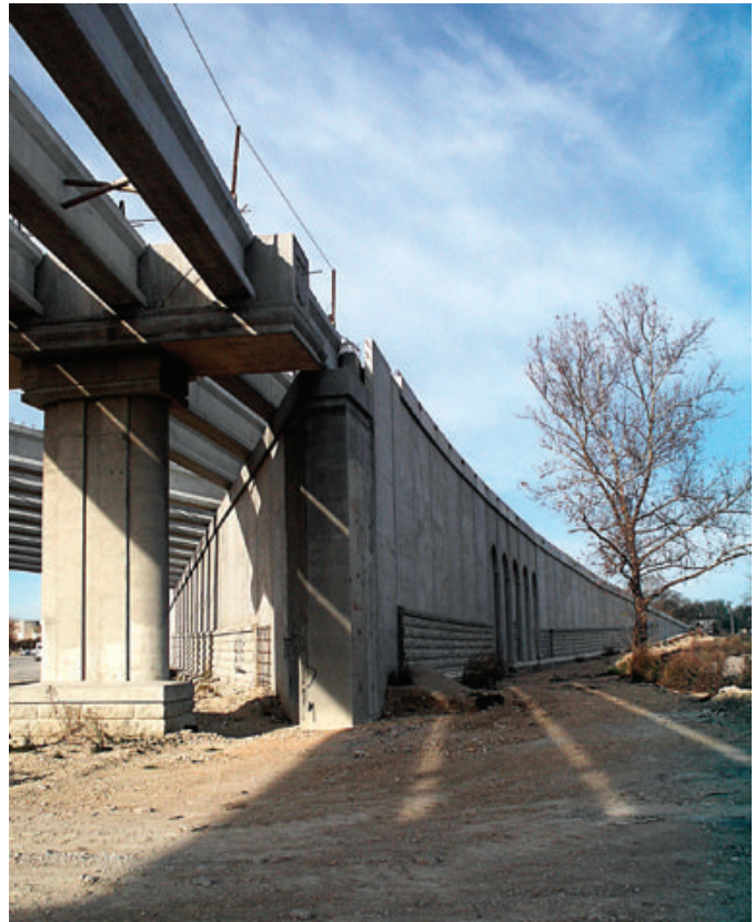
Fig. 5: Military Highway overpass at IH 410 in San Antonio, TX
