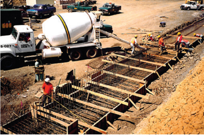
Fig. 3: Ready to place concrete in the CPC wall footing along SH 190 in Dallas, TX
