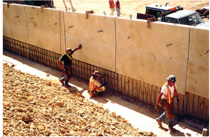
Fig. 4: Splicing flexural reinforcement to footing dowels in Dallas, TX
