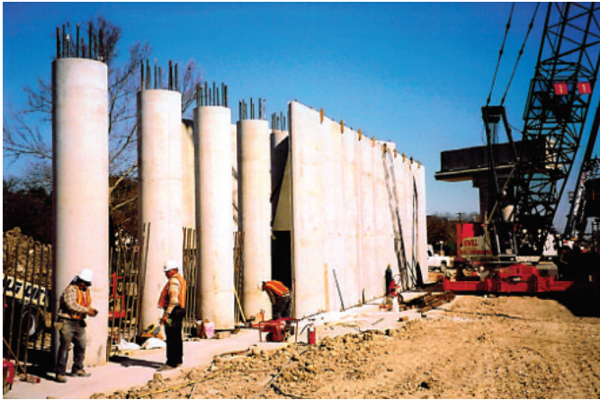
Fig. 6: Installation of CPC adjacent to drilled shafts at IH 410 in San Antonio, TX
